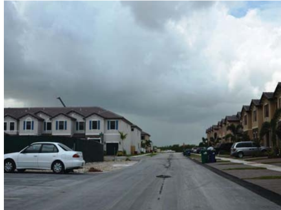
Roads, Drainage, Water, Sewer in Townhomes Area
