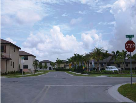
Roads, Drainage, Water, Sewer in Single Family Homes Area
